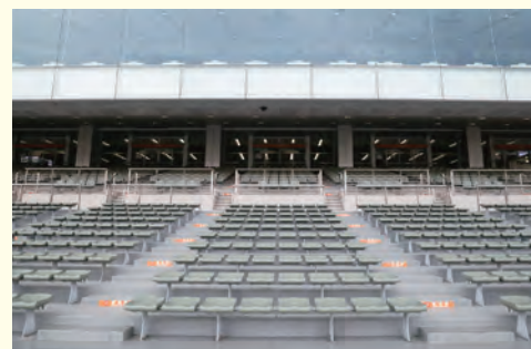
L-WING 1F Roofed seats ensure safe race watching even on rainy days.
